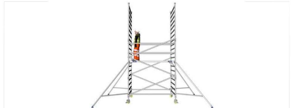
1.29 Clip the diagonal braces into place.
