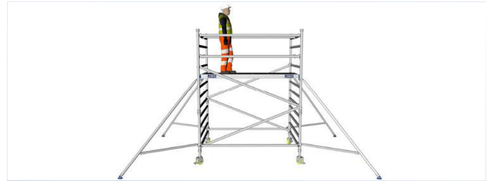
1.28 To continue building higher, fit the next set of frames on either side.
