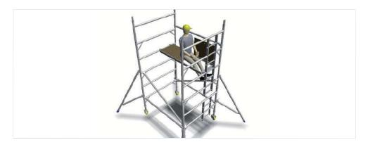
**1.21** Climb ladder and open trapdoor. Sit with feet through the platform with both feet on the ladder. Fit four guardrail braces on the 4th & 6th rungs directly above the sides of the platform.
