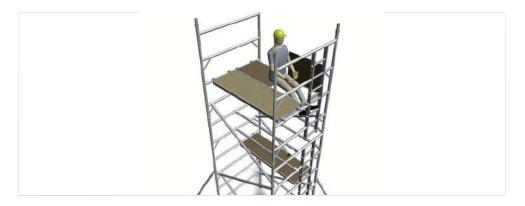
1.36 Climb ladder and open trapdoor. Sit with feet through the platform with both feet on the ladder. Fit four guardrail braces on the 9th & 10th rungs directly above the sides of the platform.
