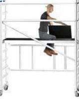
Fit the toe boards into place, then the erection of the LEWIS 1.6m 1.14 platform height Miniscaff is complete.
